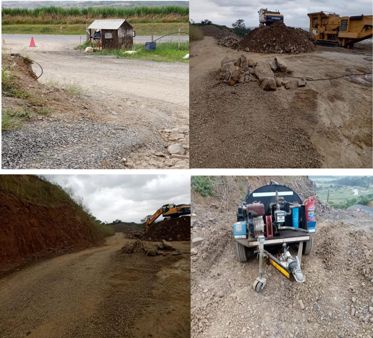
Figure 12: Mining licence Compliance Audit at Quarry mining sites eThekweni municipality
