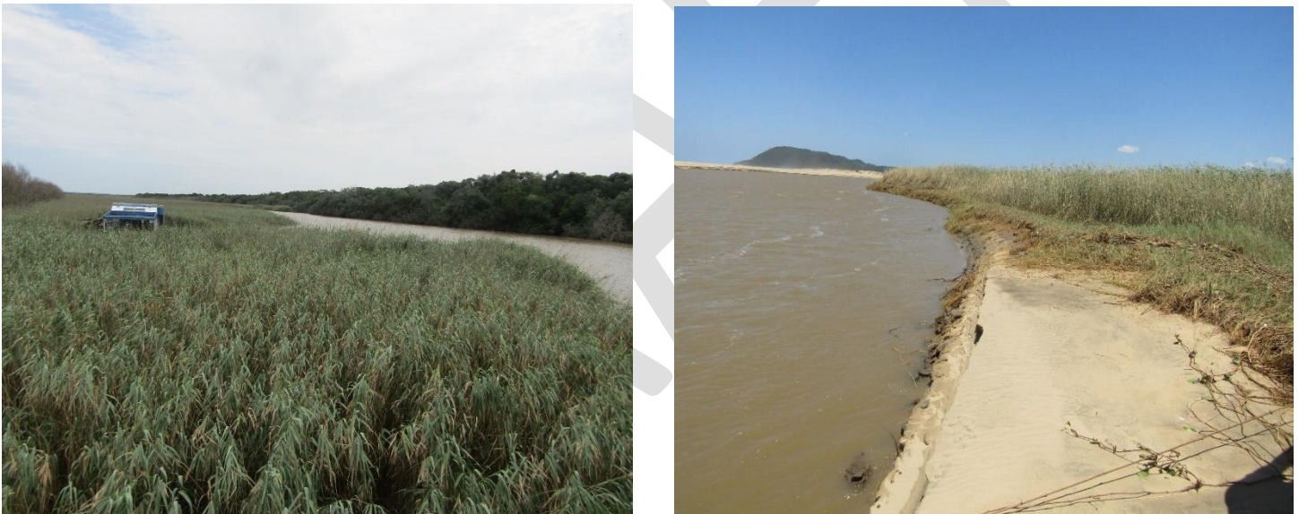
Figure 16: Reed encroachment at the St Lucia bridge and estuary mouth
